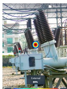
Partial discharge inspection
