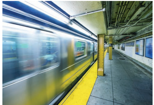
Figure 6 – Train platform and train way
