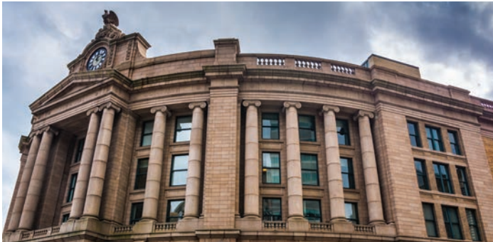
Figure 1. Boston South Station
